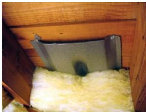
*Rafter vent—in gray above—installed between rafters where the roof meets the attic floor.*
